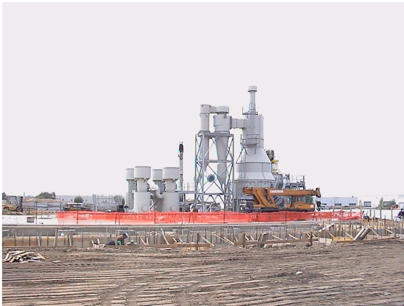
PRME 4.0MWe Biomass Fired Engine Generator System
