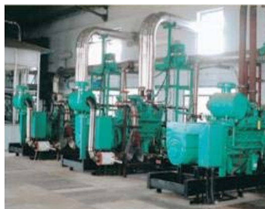
Figure 1. 100% producer gas engines at 1 MW power station in Tamil Nadu State (Source: http://mnes.nic.in/annualreport/2004-2005_English/ch7_pg4.htm )
